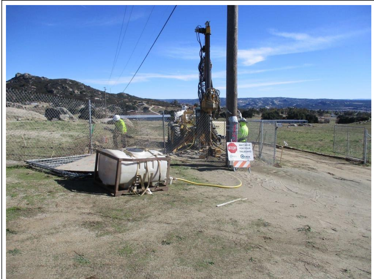
Photo 1: During perforation drilling at Pole Z46589 (TL 6923), the crew was observed using water to minimize dust emissions in accordance with APM AIR-02 and APM AIR-05.
