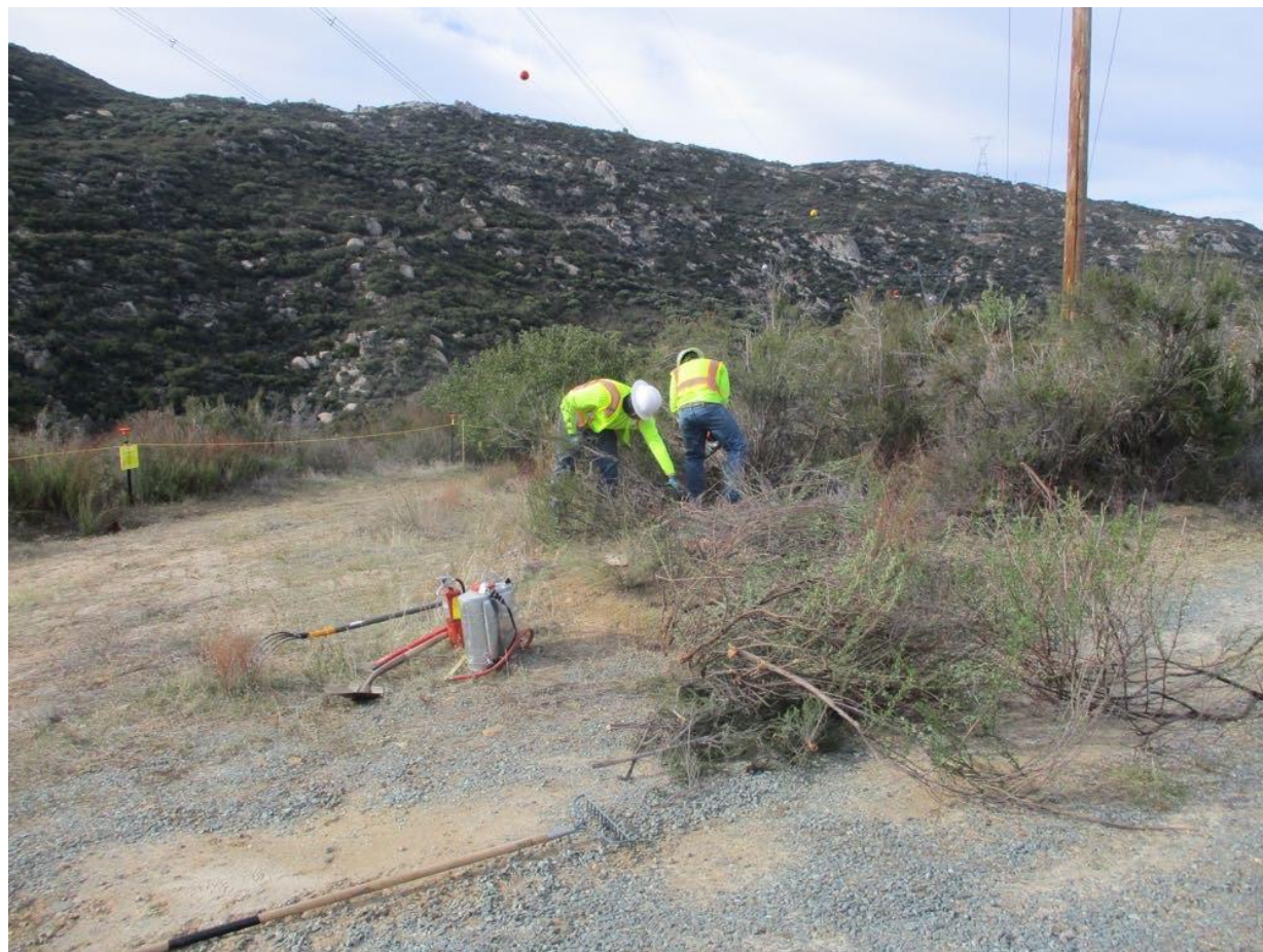
Photo 4: A vegetation removal crew at Pole Z972870 (TL 6923) was equipped with a full set of fire tools (5-gallon backpack pump, round point shovel, Pulaski, and 2A10BC fire extinguisher) within 50 feet of the activity in accordance with APM HAZ-04 and the CFPPP (MM FF-1).
